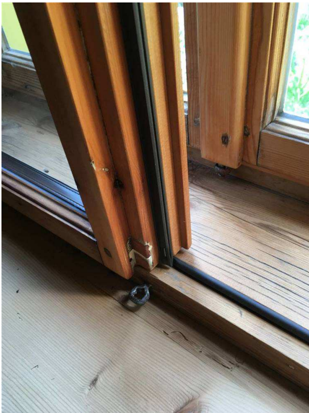
Box-type window after retrofit, detail with sealant, Darius Richter
