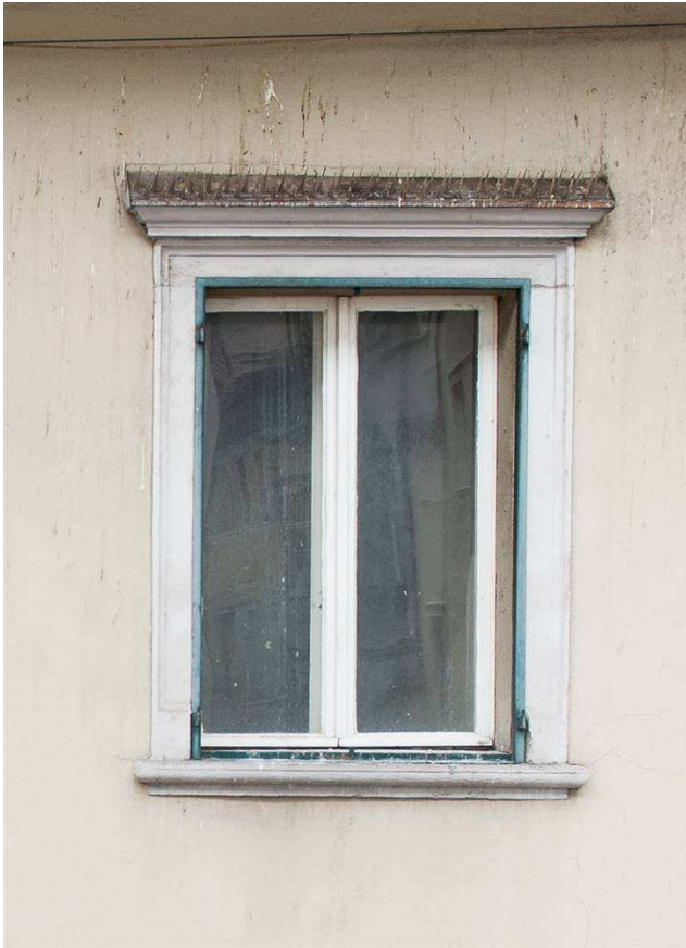
Box-type window from 1950th/60th (before retrofit), EURAC
