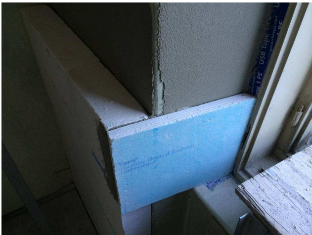
Internal insulation at the window reveal
