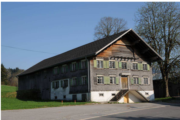
Photo of the building before the renovation, ©EIV
