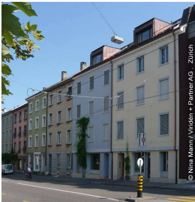
Street elevation after renovation. © Nina Mann
