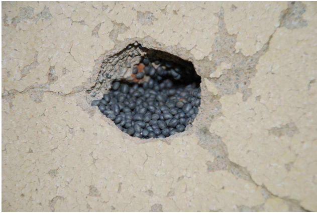
Double-shell blowing system with Isofloc H2Wall © M. Hutterli
